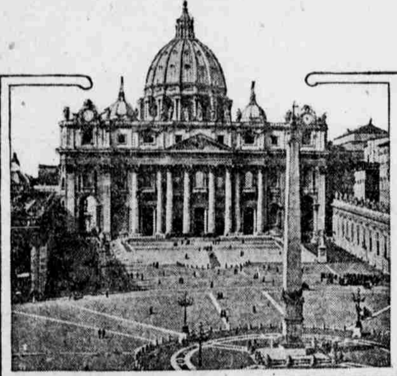
St. Peter's square in Rome was hard hit by the earthquake. The obelisk seen in the foreground in the photograph, was shaken and badly damaged; the famous colonnade, seen at the right, was lowered four feet, and the adjacent house, once occupied by the sisters of Pope Pius X, was seriously cracked.
