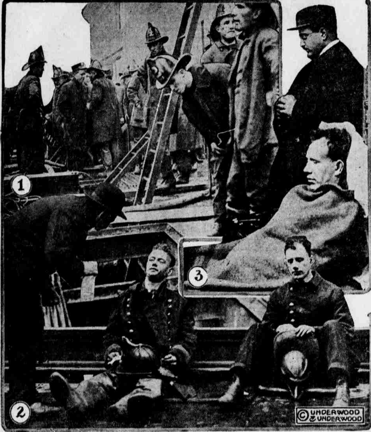
The burning of two large electric cables in the New York subway resulted in the partial asphyxiation of hundreds of passengers, and a panic ensued in which scores were injured. One woman was killed. 1. One of the gratings through which many passengers were rescued. 2. Firemen who were dragged to the street after being suffocated. 3. One of the overcome passengers lying on the sidewalk while a pulmonologist is being prepared.
