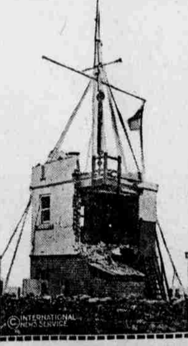
The coast guard signal station at Whitby, on the English coast, made a good target for the gunners of the raiding German warships and its condition shows their aim was excellent.
