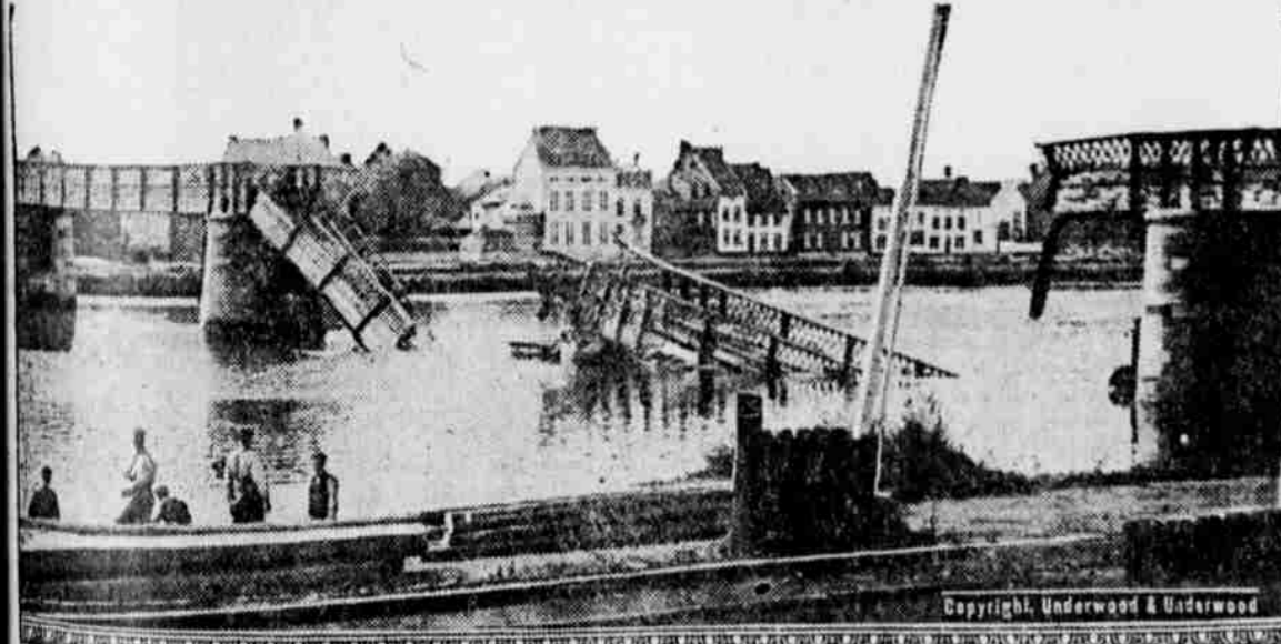
In order to impede the advance of the Germans the Belgians destroyed this steel and concrete bridge across the Meuse river. This photograph was made at great risk, as an order had been issued to shoot photographers caught making pictures.
