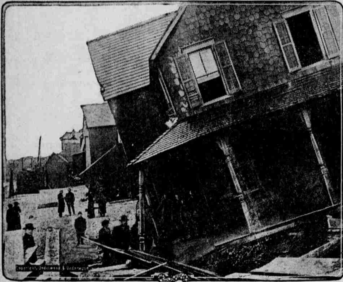
A view of the ocean front at Sea Bright, N. J., showing the wreckage left in the wake of the angry sea, which was lashed into a fury by a 95-mile hurricane that almost destroyed this summer resort on the Jersey coast. Enormous damage was caused by the undermining of the foundations of residences, which resulted in the almost complete destruction of the homes, sending hundreds fleeing into the streets, poorly clad to withstand the biting winds.
