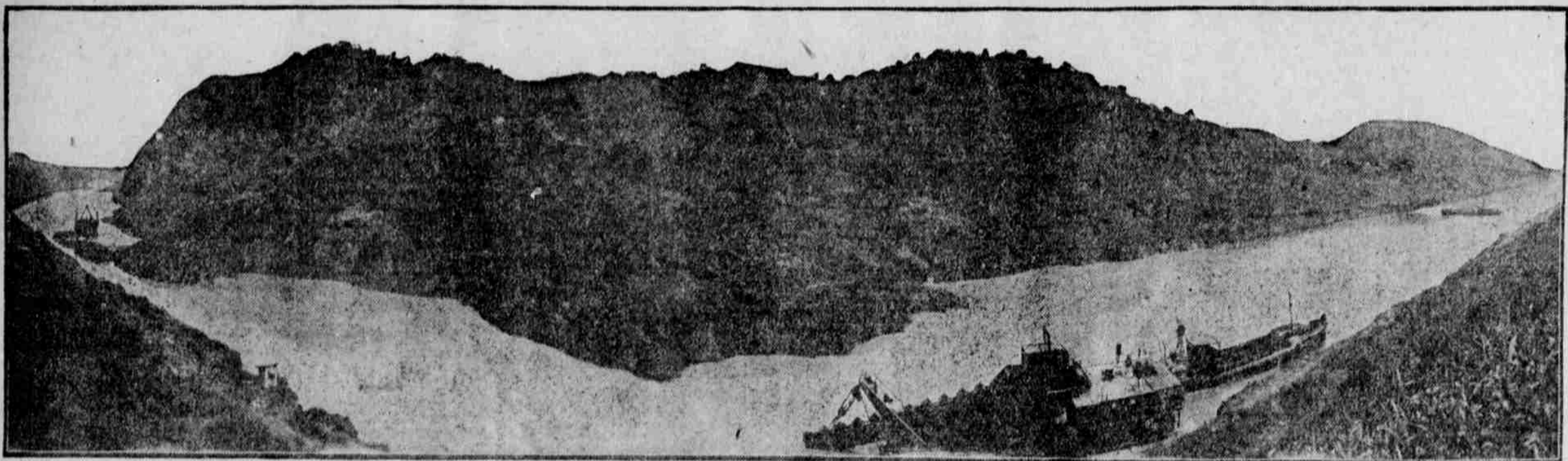
This remarkable photograph, just received from the Isthmus, shows the present condition of the Cucaracha slide in the Panama canal and the dredges at work cutting the channel through it. At the left is seen Gold hill, to the north, and at the right the canal stretches off toward the Pedro Miguel locks.
