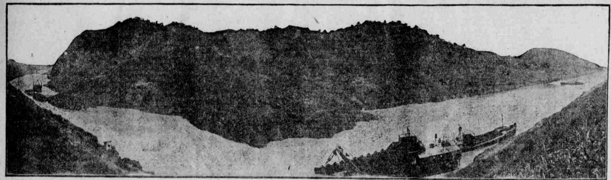
This remarkable photograph, just received from the Isthmus, shows the present condition of the Cucaracha silde in the Panama canal and the dredges at work cutting the channel through it. At the left is seen Gold hill, to the north, and at the right the canal stretches off toward the Pedro Miguel locks.
