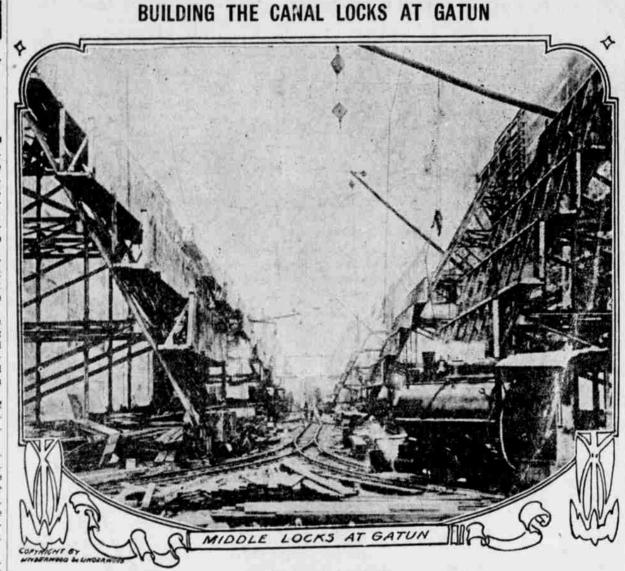
THE stupendous nature of the work of constructing the Panama canal is well illustrated by the accompanying photograph, just received from the Isthmus. The view is taken from the north end of the middle locks at Gatun. It shows the middle and upper locks and also the steel monolith forms, the latter in position to receive concrete for the middle and east wads
