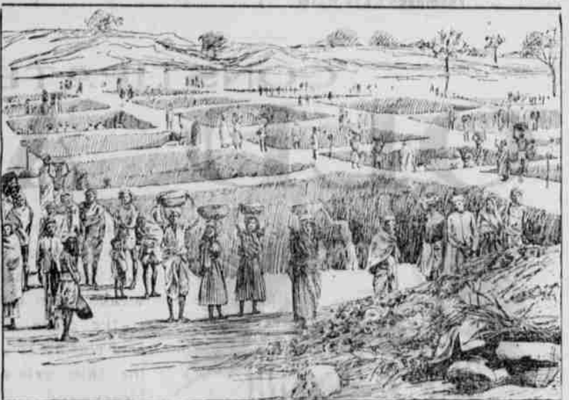
GOVERNMENT RELIEF WORK—MAKING A RESERVOIR.
