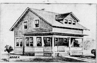
nomical, is its use for the exterior | side in the central part of the struccoating over lath. Color effects can be produced to harmonize with any desired tint of the wooden trim, by the addition of mineral coloring matter to the cement before it is mixed. Then the surface may be either trow eled smooth or may be given a rough pebble dash finish.
