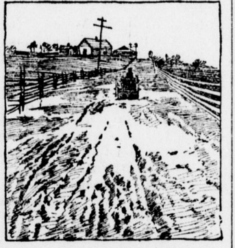
Improvement of Roads Adds to the Value of Real Estate.
