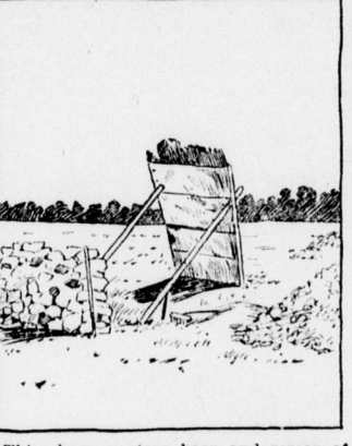
This shows a stone heap and screen of a road repairer in France. After the large stones are broken they are delivered at the roadside in regular heaps, inspected and measured. The screen protects the workman from the sun.
