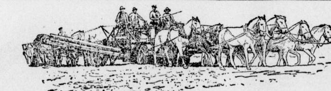
ELEVATING HORSE DRAWN GRADER AT WORK.
