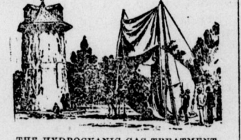
THE HYDROCYANIC GAS TREATMENT.
