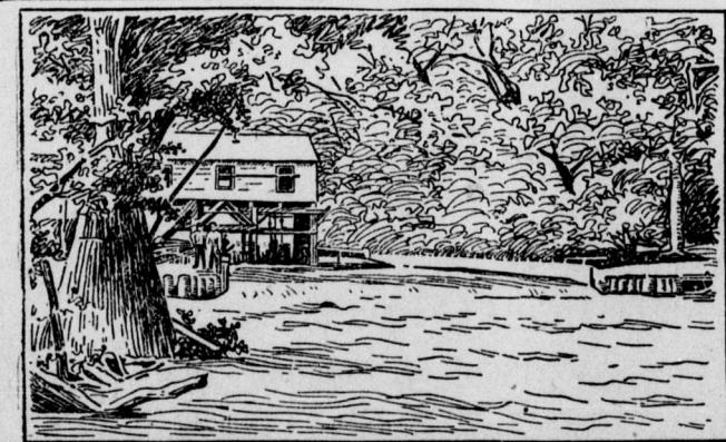
PUMPING PLANT FOR RICE IRRIGATING CANAL.
