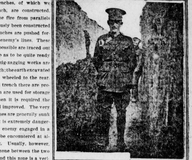
THE DEPTH OF A COMMUNICATION TRENCH (compared with the height of an officer)
