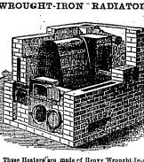
These Heaters' are made of Henry Wrought Iron, ell rivited together, the only sure prevention ainst the scape of Gas or Dust. They are oasily anaged, without any dampers: The Patent Rador avoids the use and aunoyance of drums, and permanen'ly attached to the Heater. This is most dirable, simple, euconomical and popular acting Apparatus ever offered for sale. They are I guaranteed.
