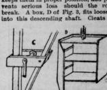
FIG. 3.-WELL BOX AND WINDLASS. side with movable shelves fit it for holding any size of cans, jars, etc. A door closes the front, and a three rope The rope is first tied to the ring above this pulley, taken up over one of the pulleys at A. Fig. 2, down beneath the pulley on the box, up over the second pulley at A, back over pulley B, and down to the windless.
