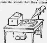
A, represents the funnel; B, the phonograph; C, the kinetograph, and D, the electric battery.
