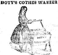
which is rapidly becoming popular and with this Machine the hard work of washing is mitigated to a comfortable and pleasant task. The clothes are placed in hot suds, and shut in. While thus immersed and the steam confined, the Machine is operated as seen above. Thus the work is speedily, clearly and easily done, and that too without tearing and wearing out the clothes, which to a great extent is the cause under the old fashioned rubbing process With a
