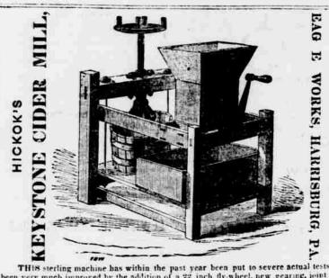
THIS sterling machine has within the past year been put to severe actual tests, and been very much improved by the addition of a 22 inch fly-wheel, new gearing, joint bolts, and other minor improvements, and is now offered to the public with the certainty that it is made in the very best manner, and that it will grind and press casier and faster than any other Mill in the market. Dealers and others supplied on liberal terms.
