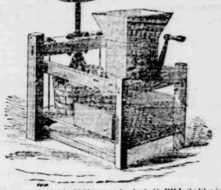
I N the present arrangement of this highly approved and valuable MILL, the labor is divided by arranging a cutting Cylinder to break the apples, and then deliver them to the lower cylinder to be reduced to pomace. By this arrangement the work is performed faster and with much less Inbor.
