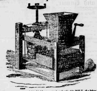
N the present arrangement of this highly approved and valuable MILL, the labor is divided by arranging a cutting Cylinder to break the apples, and then deliver them to the lower cylind to be reduced to pomace. By this arrangement the work is performed faster and with much i Will commence on Mospar, Ocroses 17th,
