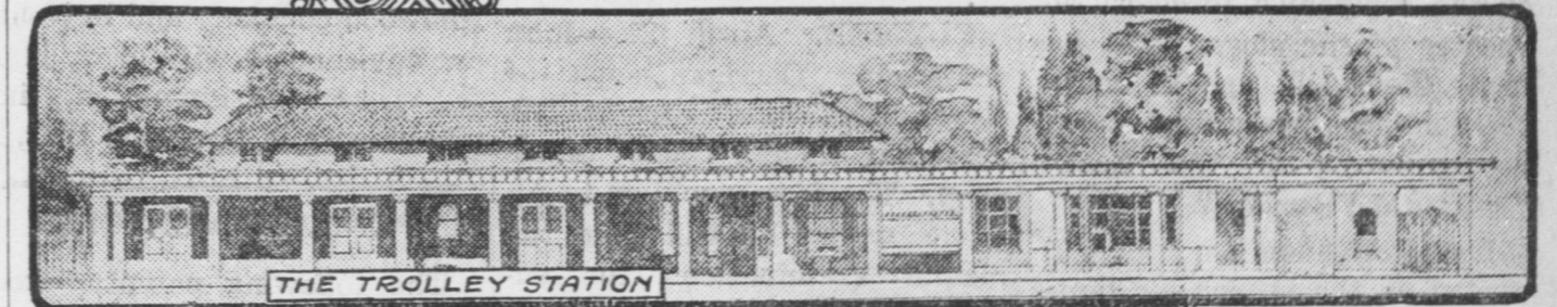
THE TROLLEY STATION
