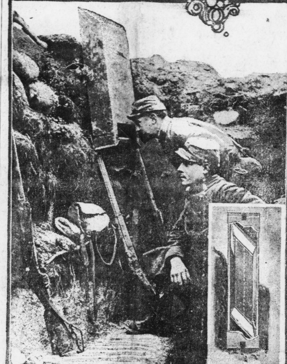
Photo by American Press Association. Simple arrangement by which the soldiers can see what is in front without exposing themselves to fire.
