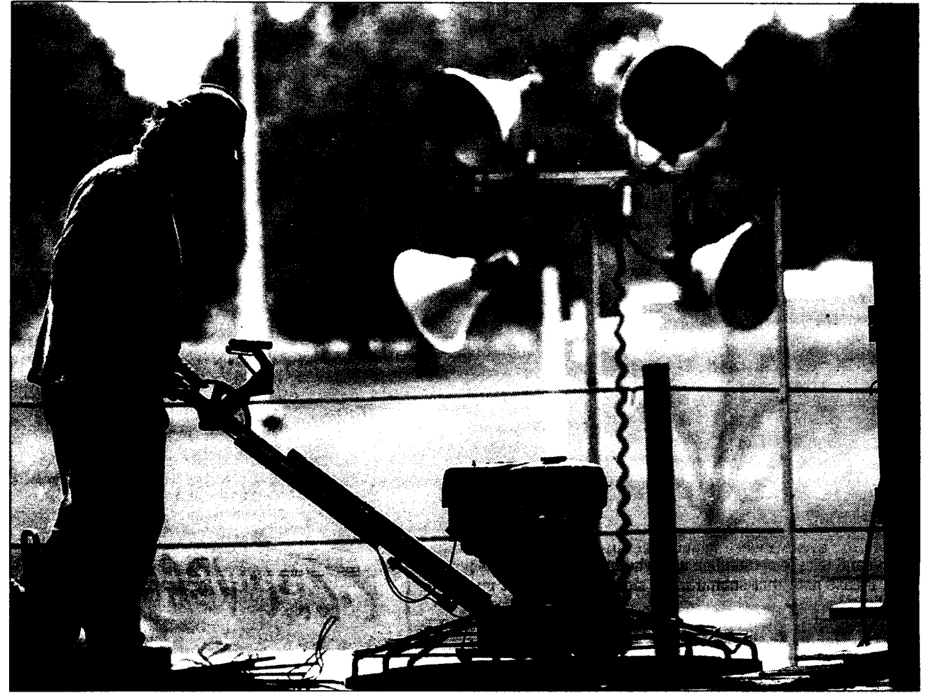
POURING IT ON: Kenny Nepp, a worker with Mountain Top Concrete, smooths over freshly poured concrete on the second floor of the Information Sciences and Technology Building. Construction is expected to be completed by Fall 2003.
