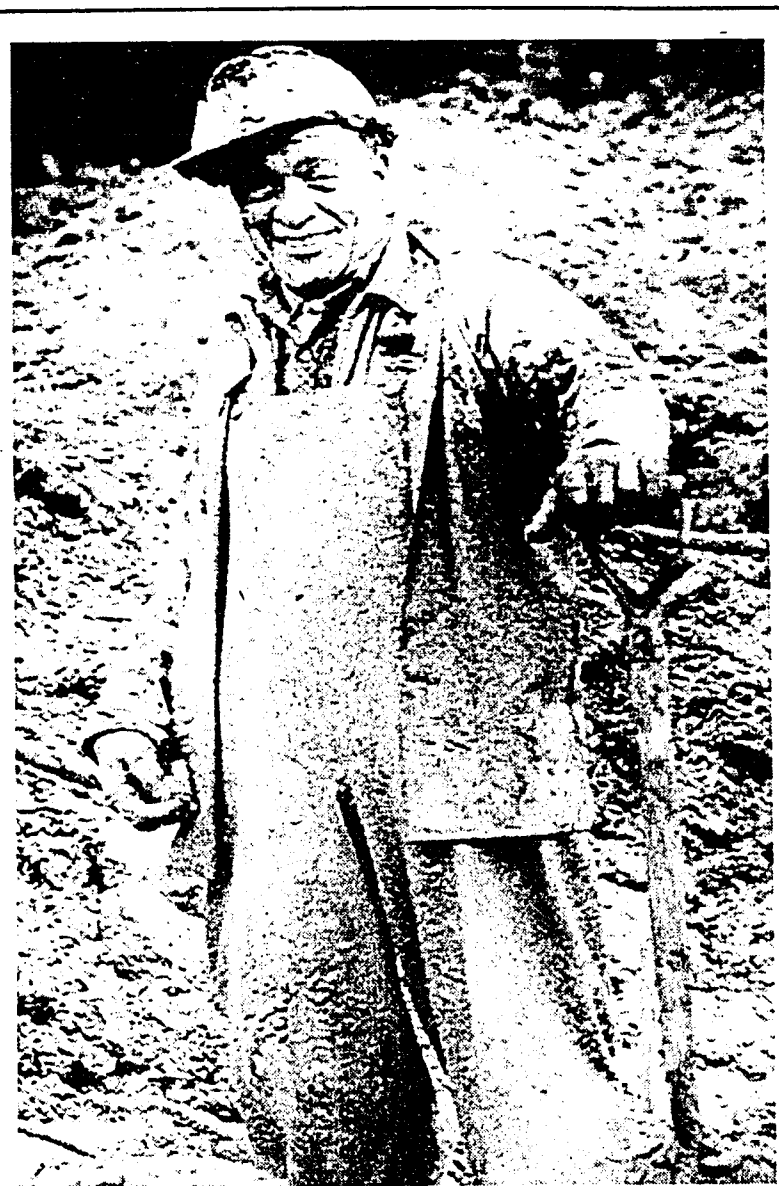
Mudman Construction worker Lonnie Boyd emerged from the depths after braving wind and rain during the building of two towers in downtown Durham, N.C. this week.
