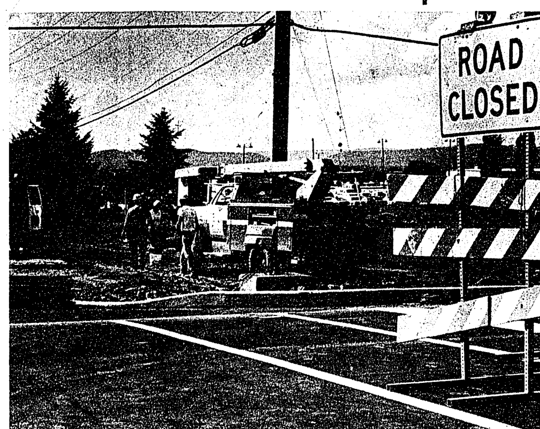
Workers oversee construction that has been taking place all summer at Park Avenue and Bigler Road.
