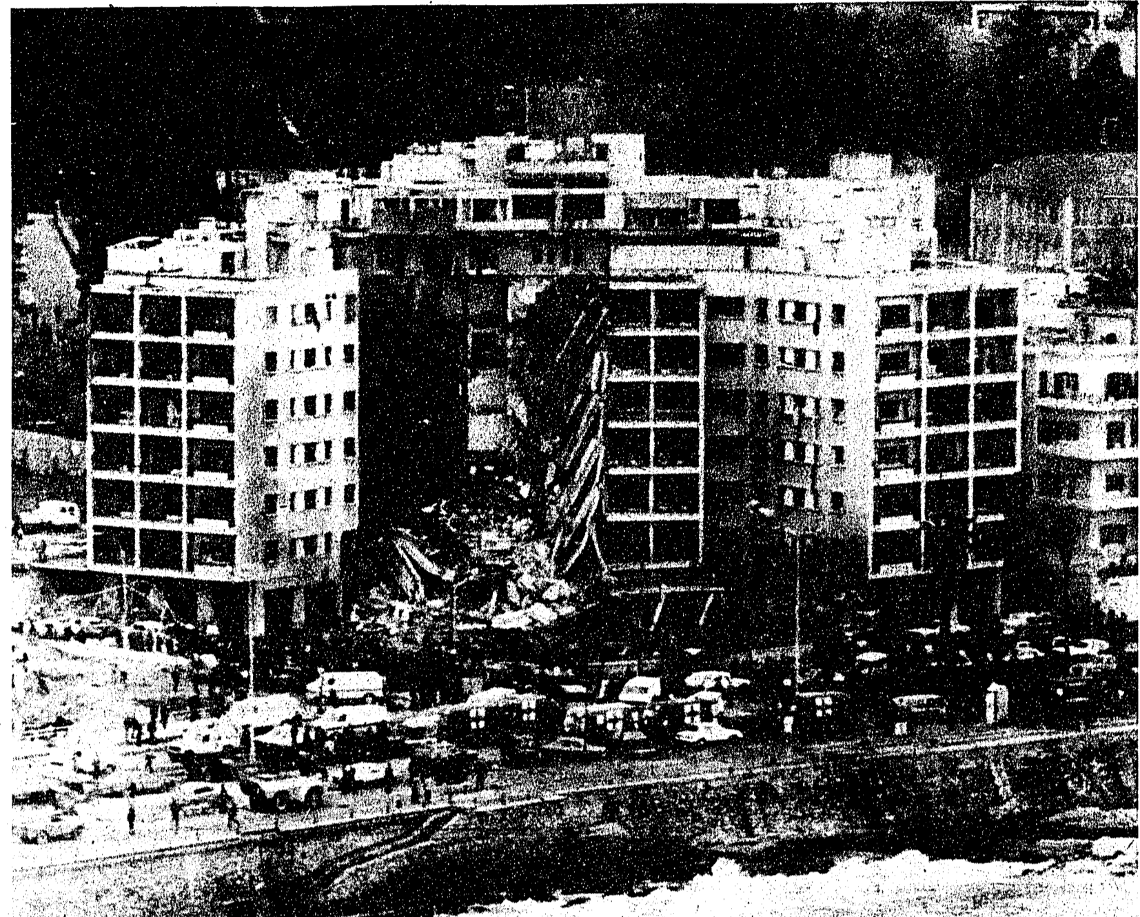
An aerial view of the U.S. Embassy in Beirut shows damage done after a bomb exploded outside the building Monday. There have been 24 confirmed deaths, including eight Americans, resulting from the blast. Twenty-three people are still missing.
