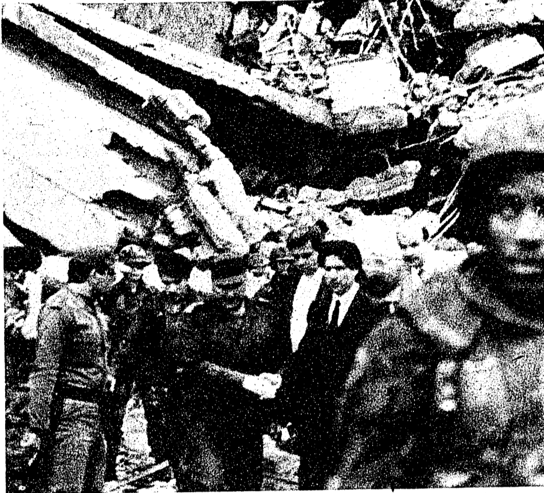
Lebanese President Amin Gemayal shakes hands with Lebanese Army Commander General Ibrahim Tannous yesterday as they view the damage at the U.S. Embassy in Beirut after a huge bomb went off collapsing the entire facade of the seven story building and killing 39 people.
