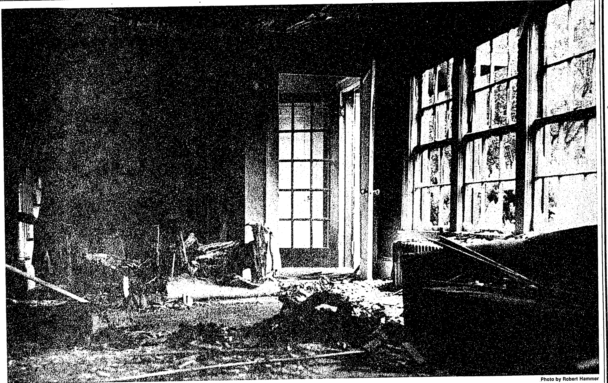
Fire and smoke caused extensive damage to this house at 525 S. Pugh St. yesterday. Police have not determined the cause of the fire.
