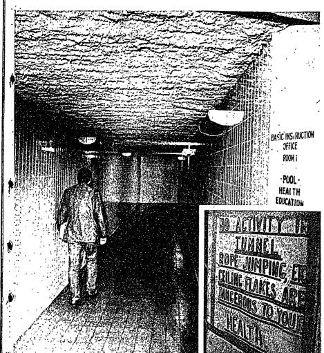
Flaking of asbestos surfaces, a possible cancer hazard, is seen here on the ceiling of a hall in White Building. Though no hazard has been established to exist, warning signs have been posted to decrease the possibility of producing asbestos dust which might be dangerous if inhaled.
