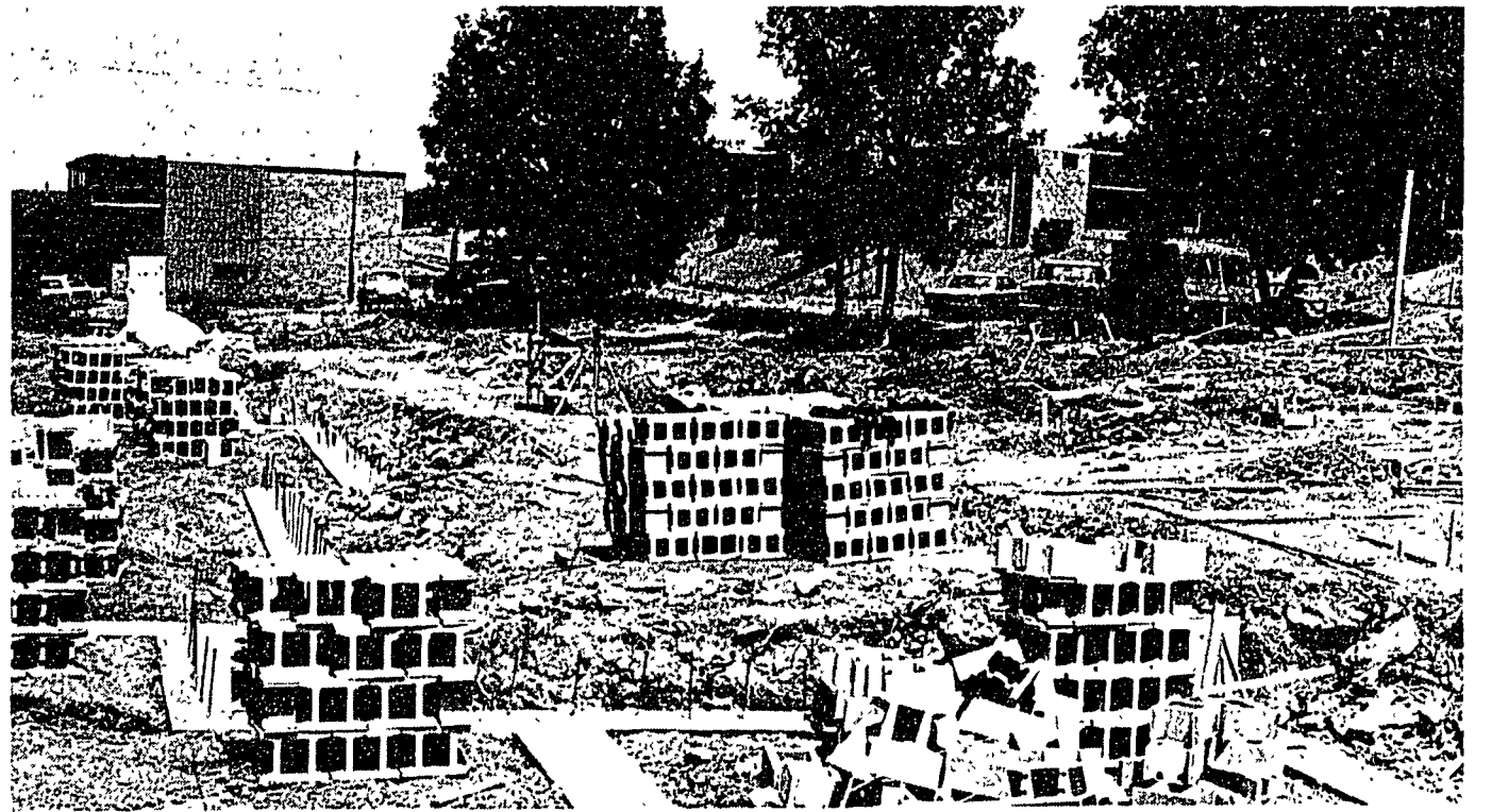
Construction has begun on the borough's senior citizens housing project on Bellaire Ave. near Eastgate apartments. Photo by Patrick Little
