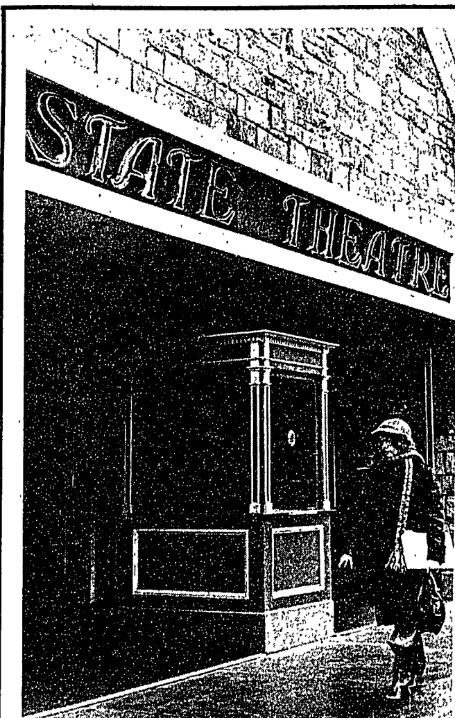
A woman walks past the closed doors of the State Theatre (right). The State was shut down by local code enforcement officers. The theatre was cited (left) for a number of violations of local building and fire codes.
