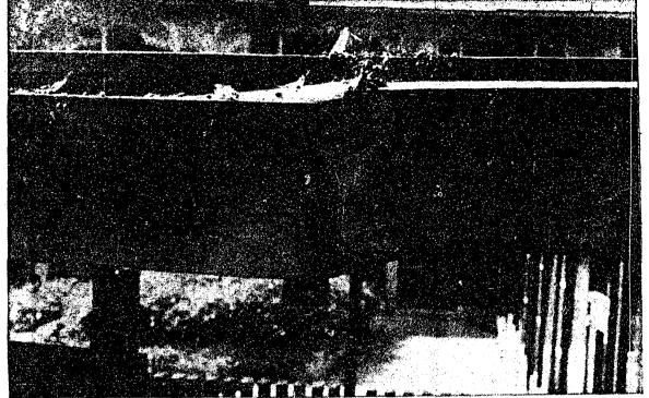
ANOTHER JOB FOR ATLAS: No, you're not seeing things-the concrete canopy in front of the Hetzel Union Building is sagging again. The condition was first noticed soon after the HUB was completed, and last year pipe column shores were installed in an effort to stop the settling. Walter H. Wiegand, head of the Physical Plant, has cited temperature changes as one of the possible causes
