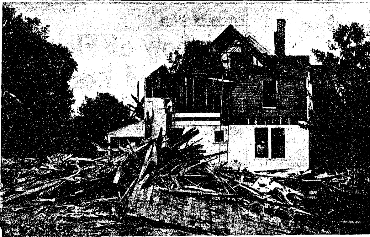
THE DEMOLITION of a house, formerly used as a boarding house, on S. Pugh St. is the end of an abode steeped in the history of freshman customs. The house, known as "The Fort," was a boarding house when the class of 1899 was going through customs. A frosh who defied customs put up a stand against upperclassmen there who attacked the residence with a Civil War cannon.
