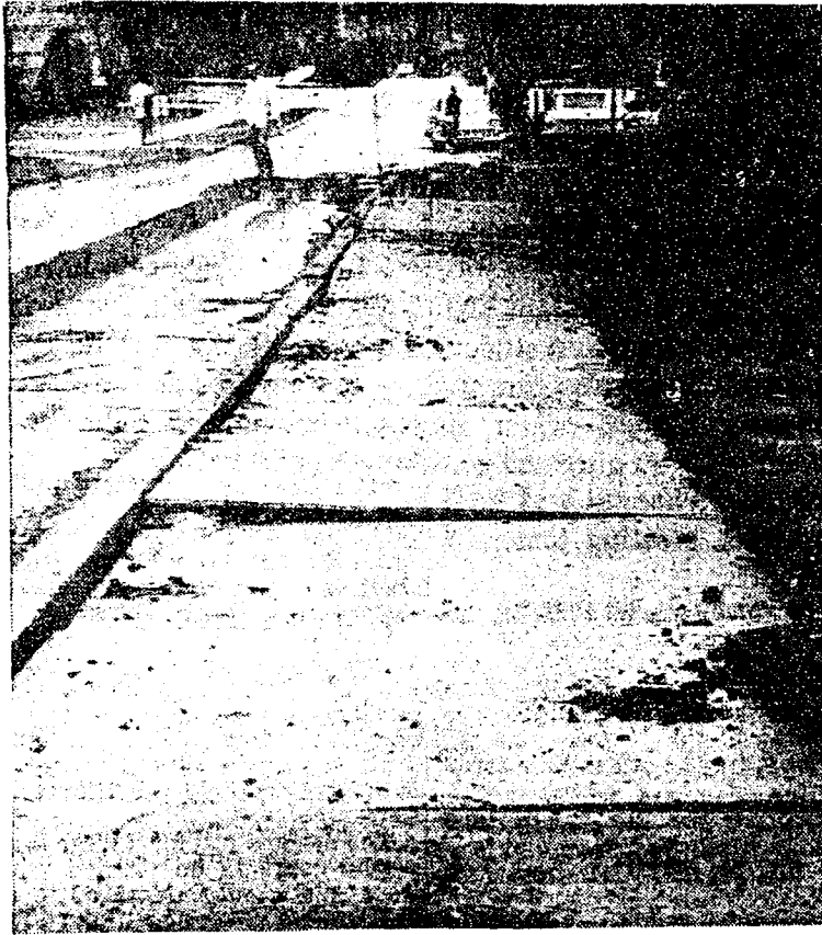
—Collegian Photo by John Beauge EVERYTHING HAS ITS UPS AND DOWNS , even sidewalks. This one, on Frazier Rd. across from Moffet Cottage, has begun to sink as the warm, wet weather thaws the frost.
