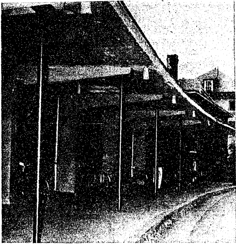
THE HUB IS FALLING DOWN??? Temporary supports have been placed on the walk in front of the HUB to help support the sagging roof. The cause of the cracks or the extent of damage is unknown, according to workmen.
