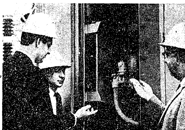
Out in the field, a company operations engineer answers questions as Serafini and Perry tour the service territory for study and inspection of equipment.
