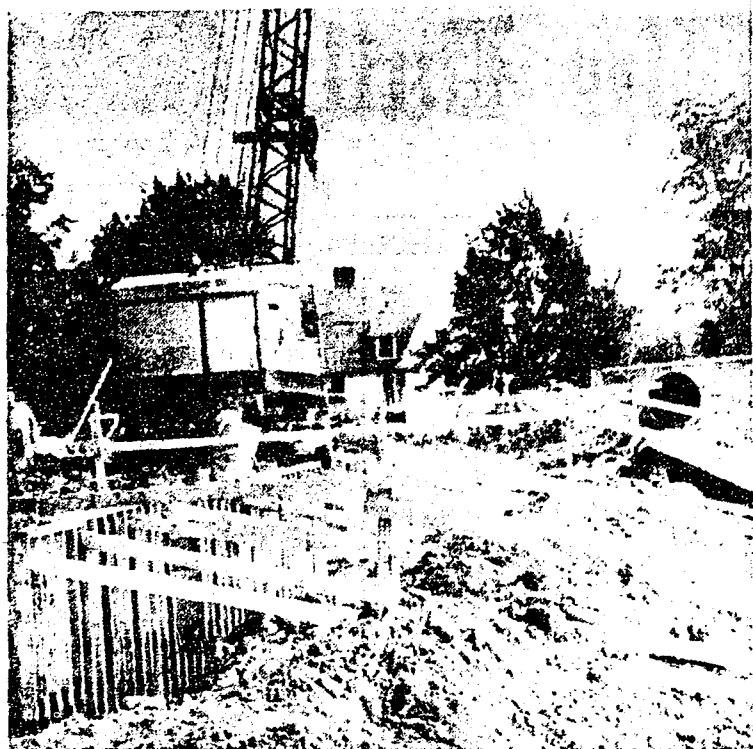
THE FOUNDATION FORMS stand like a picket fence awaiting cement. They are part of the new education building that is being built where Beaver Field used to be.
