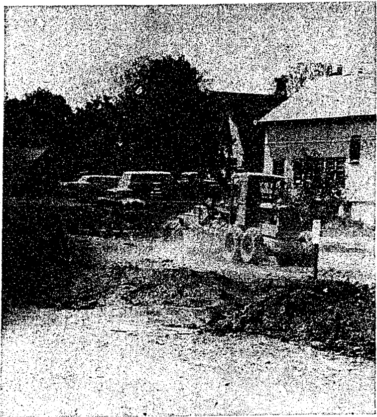
NEW PARKING AREA being prepared for student parking on corner of Curtin and Entrance Roads across from Turf Plot Residence Hall project.
