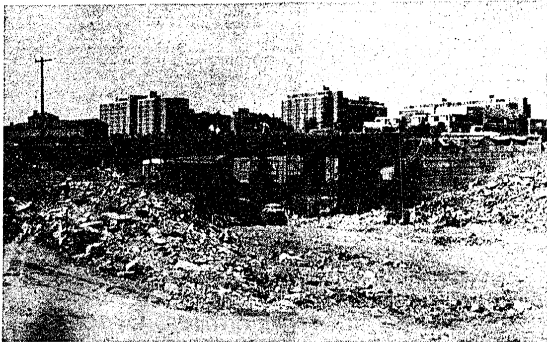
NEW OVERPASS and cloverleaf being constructed at east end of campus will be welcomed on days of future events at Beaver Stadium. The cloverleaf will connect the Benner Pike with University Drive, which will be a major artery for stadium traffic.
