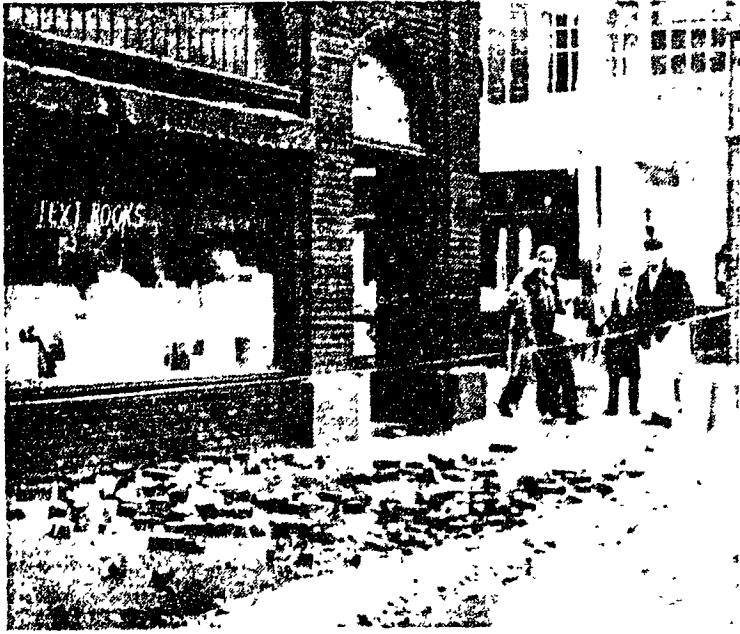
—Collegian Photo by Rick Bower BRICKS TUMBLED AND WINDOWS WERE smashed when melting snow caused part of a wall to loosen in the "A" Store Building yesterday afternoon. Two people were injured in the accident.
