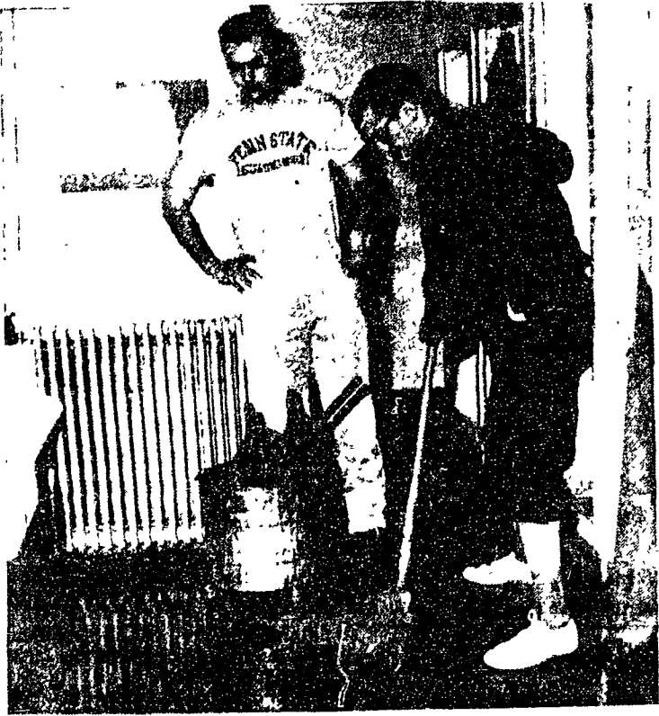
—Collegian Photo by Rick Bower WHERE ELSE BUT NITTANY —Joel Shapiro, sophomore in animal husbandry from Mt Vernon, N.Y., and Henry Fletcher, junior in chemistry from Morristown, N.J., survey the damage done in Nittany 40 when a water pipe broke
