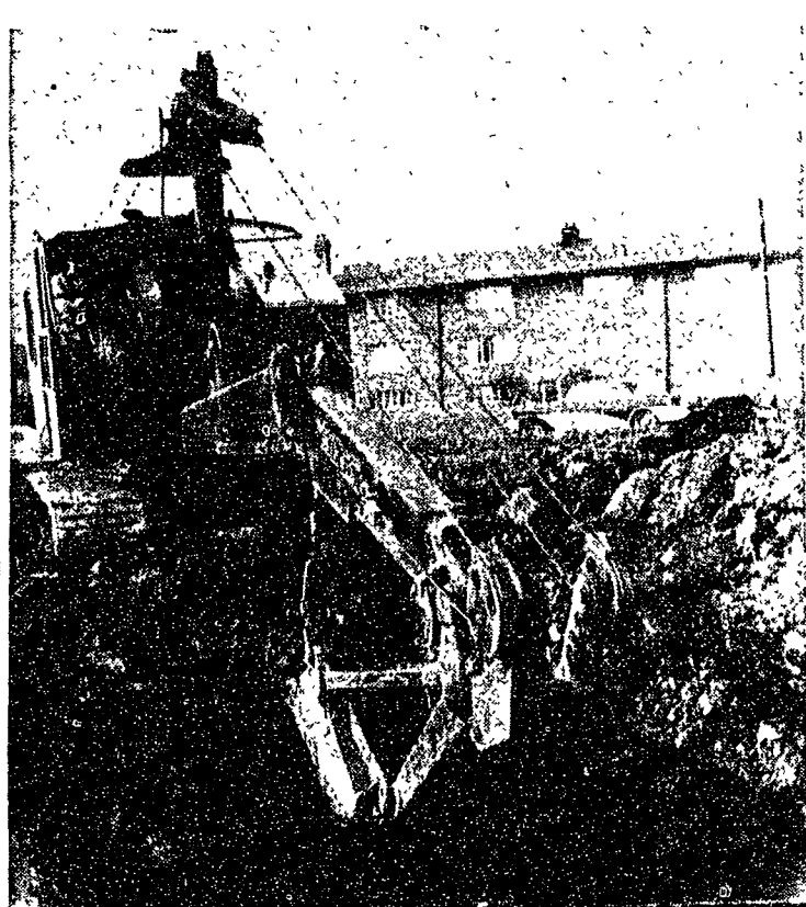
BENNER PIKE CLOVERLEAF—This backhoe moved into action yesterday as work began on the cloverleaf to connect College Ave., University Dr., and Benner Pike.
