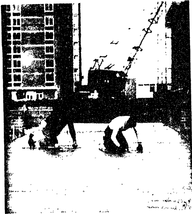
—Collegian Photo by Margie Frear SMOOTHING OUT THE LUMPS in the freshly-laid cement walks is one of the last phases in the outside construction in the new Pollock dorms. The eight new buildings in the Pollock Project are slightly ahead of their completion schedule.
