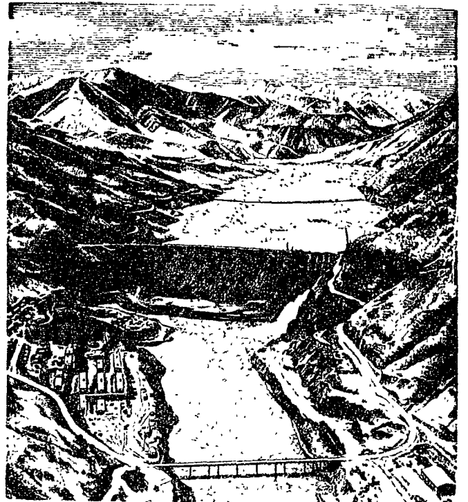
The year-old Brownlee power dam on the Snake River between Idaho and Oregon, built by the local independent electric company, the Idaho Power Company. The project embraces the Oxbow dam and the Hells Canyon dam down river from Brownlee.
