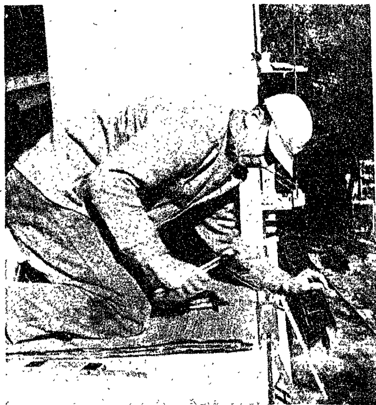
—Collegian Photo by Sam Wilson HIGH ABOVE COLLEGE AVENUE —Construction is proceeding rapidly on the Hammond Engineering Building. This worker is affixing the brackets for the siding and windows on the fourth floor.
