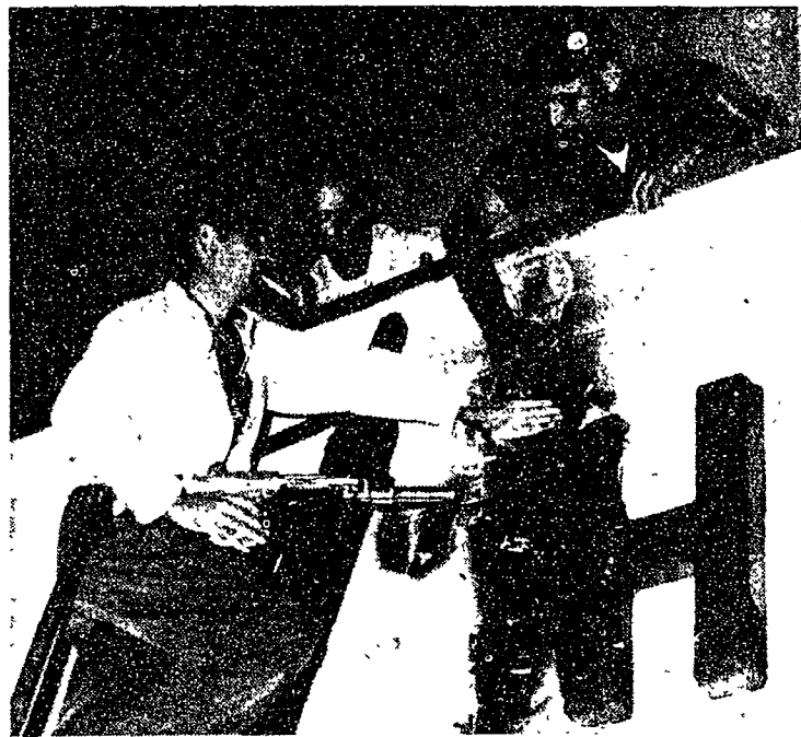
—Collegian Photo by Marty Scherr CHECKING THE DAMAGE—Alpha firemen look at the aftermath of a fire at the New Charles' Shop last night. The fire, caused by a short circuit in the sign, caused small damage.
