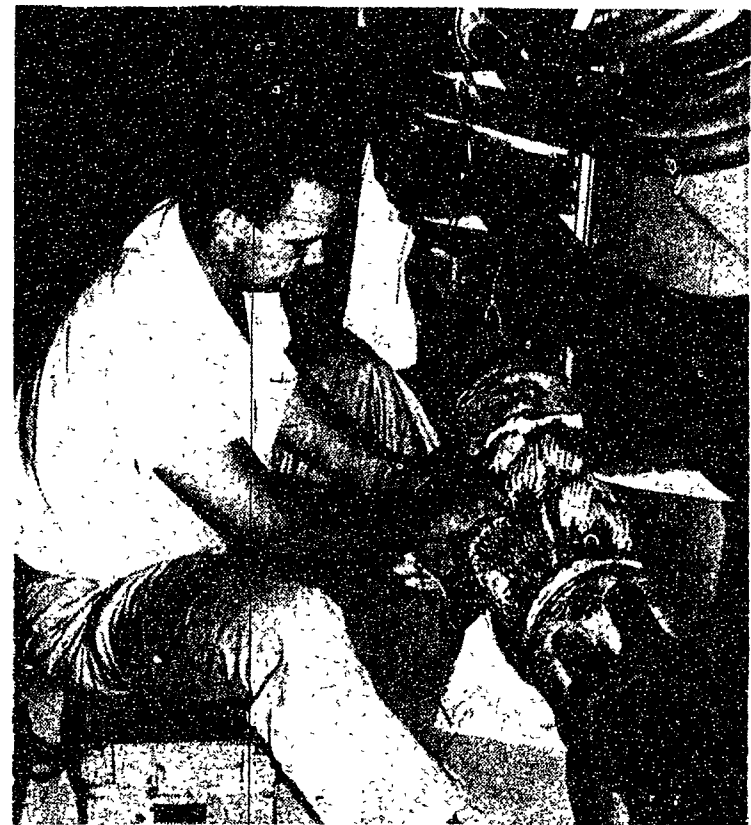
Collegian Photo by Wayne Schlegel CABLE VAULT houses 2400 pairs of wires as they come in underground from off-campus lines. A total of 9600 wires lead into the dial equipment in the new Telephone Building.
