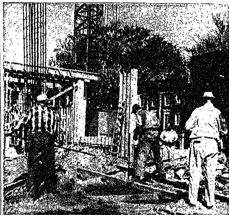
CONSTRUCTION CONTINUES on the new Hammond Engineering Building as the workers pour the concrete base. Good weather during the last week aided construction.
